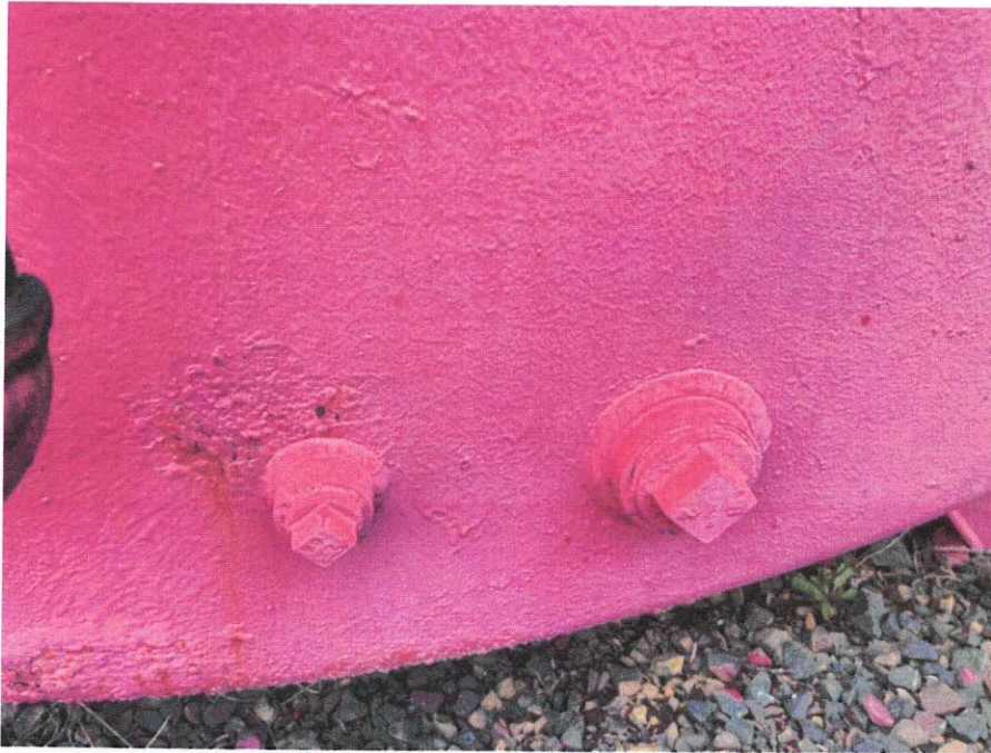
Appurtenances/IMG_8139.jpeg Isolated areas of coating failure and corrosion along tank.
