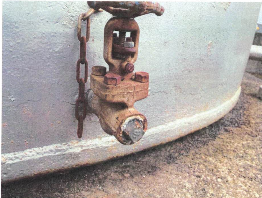
Appurtenances/IMG_8041.jpeg Coating failure and corrosion on appurtenances
