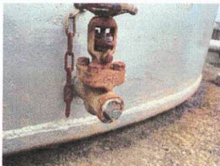
Coating failure and corrosion on appurtenances
