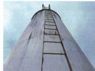
Coating failure and corrosion on ladder
