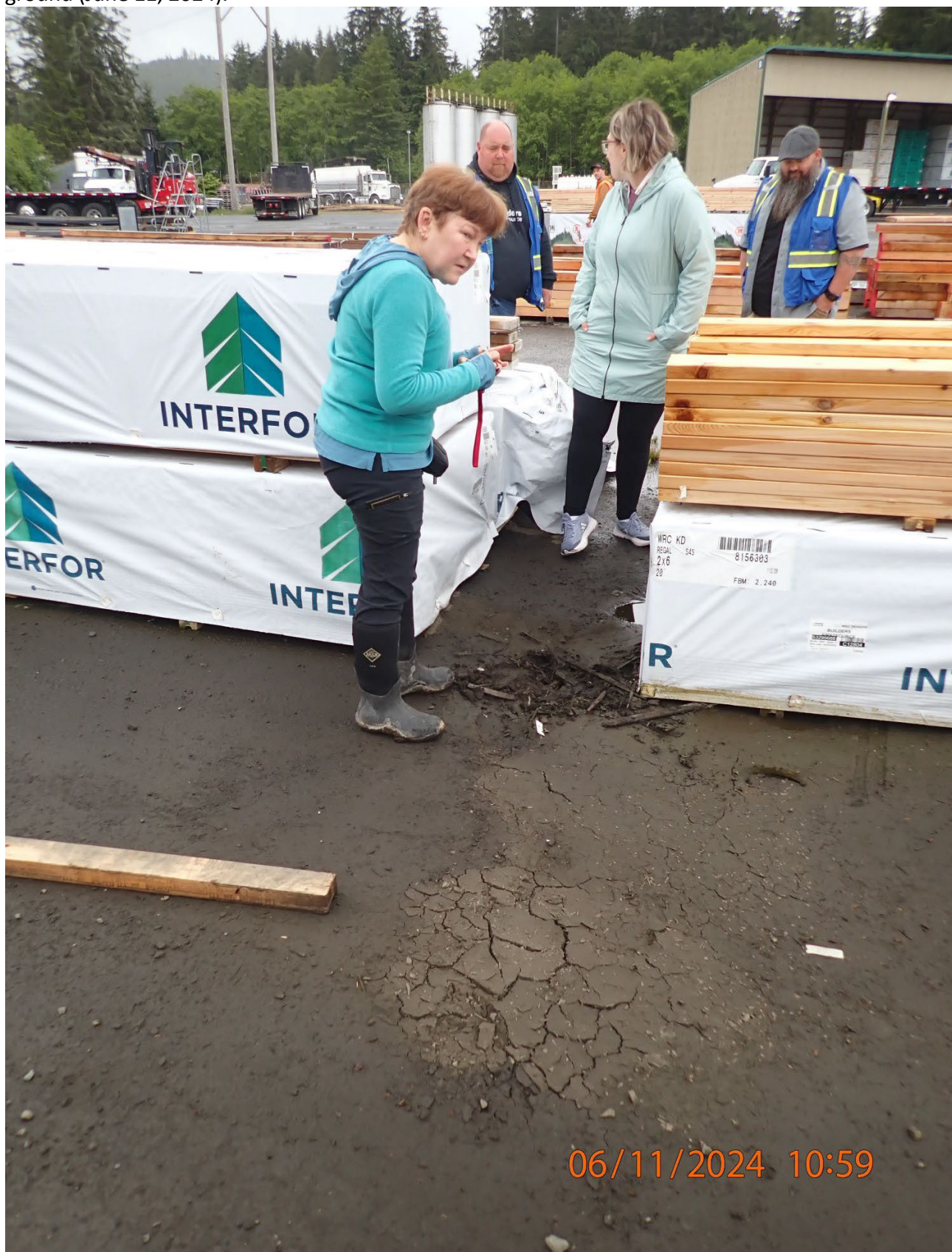
Photo 9. Storm drains within the lumberyard are filled with sediment and debris, both surficially and below ground (June 11, 2024).
