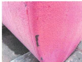
Minor coating failure on tank shell
