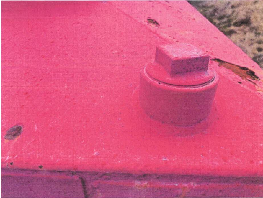
Appurtenances/IMG_8216.jpeg Minor coating failure and corrosion on shell
