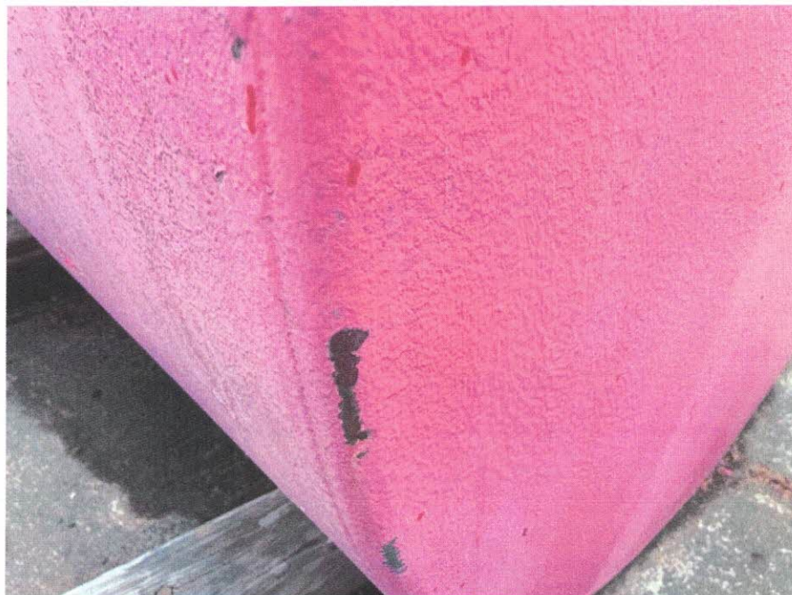
Shell/IMG_8179.jpeg Minor coating failure on tank shell
