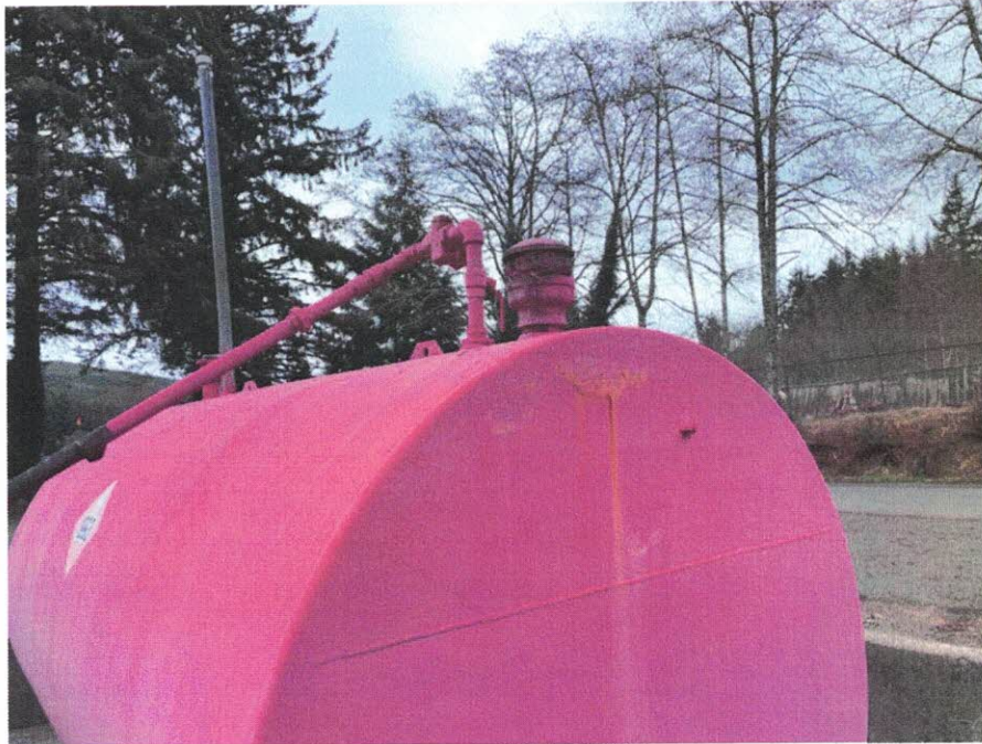
Appurtenances/IMG_8160.jpeg Isolated areas of coating failure and rusting along tank.
