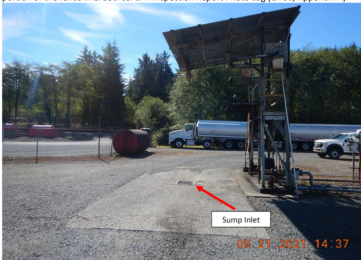
Photo 15. View, facing south, of the facility's truck loading rack. Note the lack of a raised berm along the visible portion of the fence line. Source: EPA Inspection Report Photo Log (CX 01, Appendix A).
