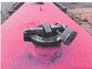
Minor coating failure and corrosion on shell
