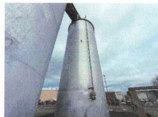
Coating failure and corrosion on ladder
