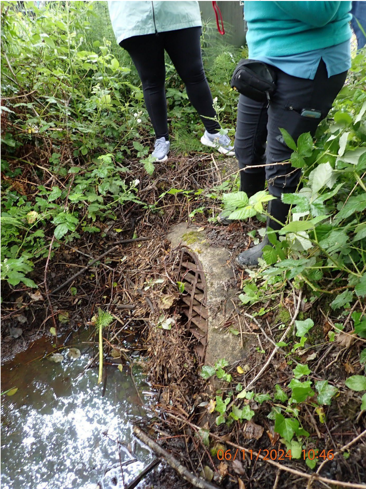
Photo 2. Inlet of stormwater culvert at the corner of lumberyard (June 11, 2024).
