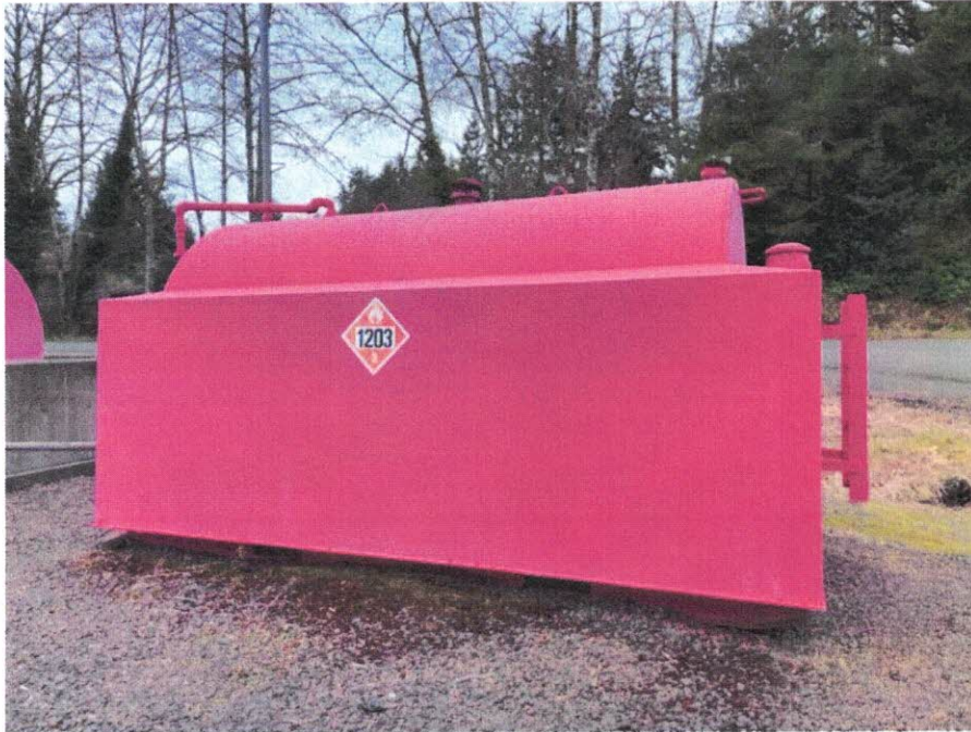
All/IMG_8192.jpeg Super gasoline tank
