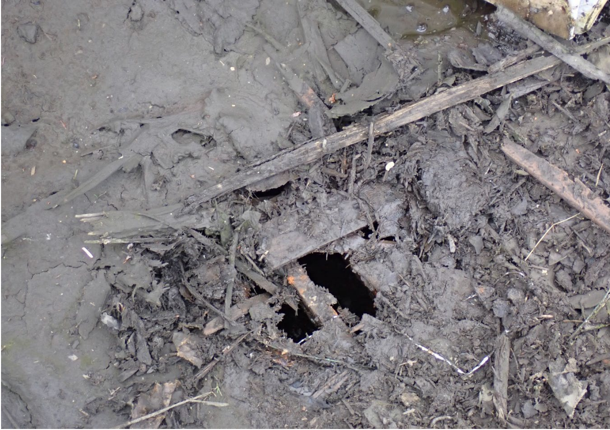
Photo 10. Closeup view of storm drain grate from Photo 9 that is filled with sediment and debris (June 11, 2024).
