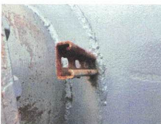
Coating failure and corrosion on appurtenances
