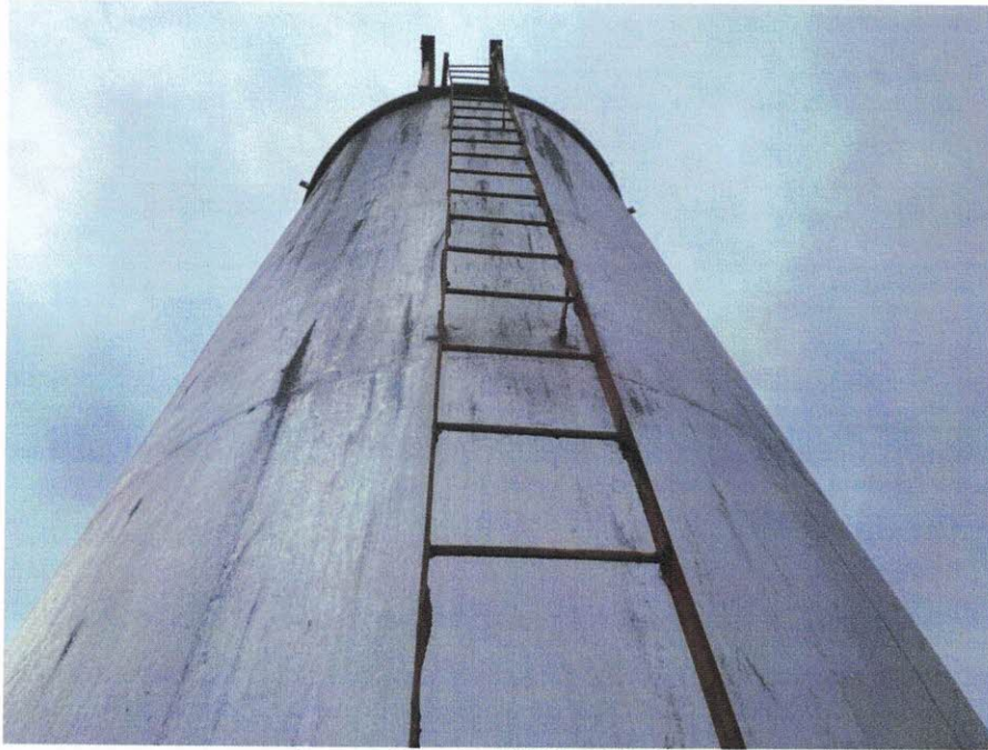
Access Structure/IMG_8067.jpeg Coating failure and corrosion on ladder
