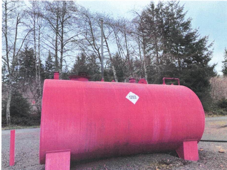
All/IMG_8115.jpeg Missing NFPA 704 Hazard Diamond,
