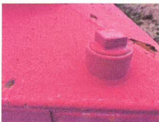
Minor coating failure and corrosion on shell
