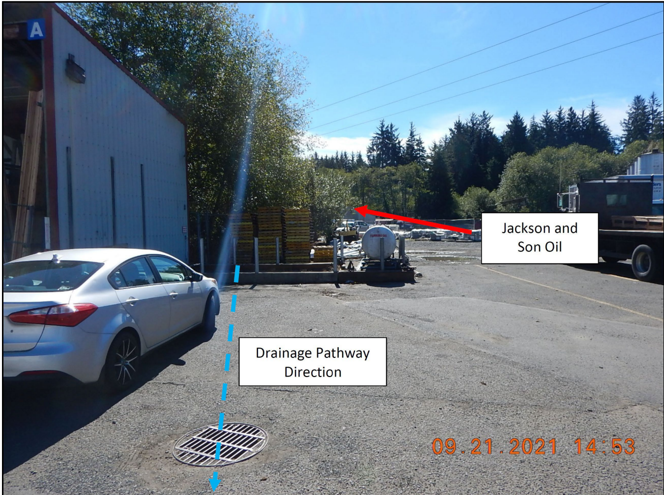
Photo 1. View, facing southeast towards the facility, of the drainage pathway from the northeastern portion of the facility. Note that the manhole inlet pictured is above the subsurface drainage conveyance running from the northeast side of the facility under the lumberyard to a wetland area located north of the lumberyard. Source: EPA Inspection Report Photo Log (CX 01, Appendix A).
