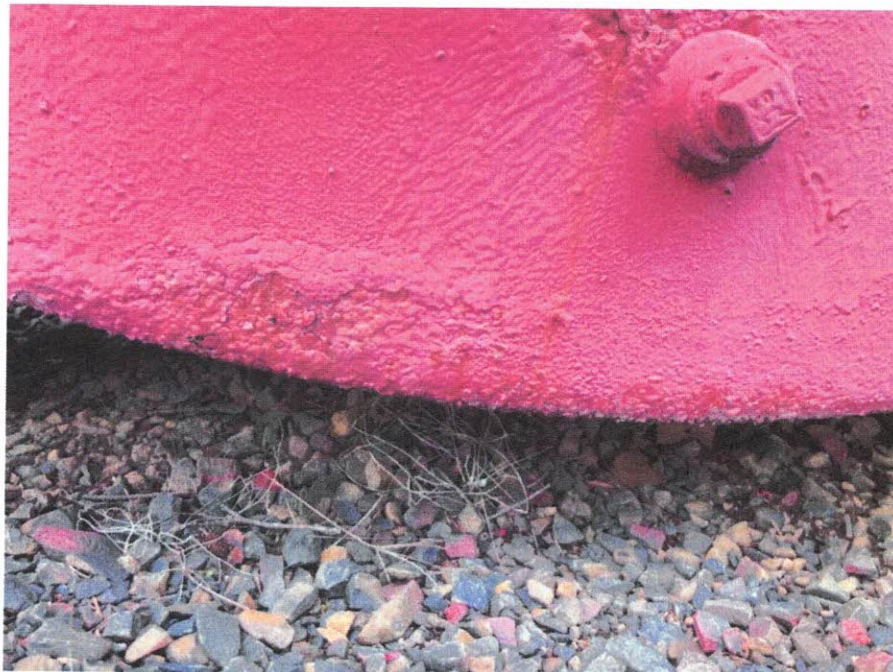
Corner Weld/IMG_8140.jpeg Minor coating failure
